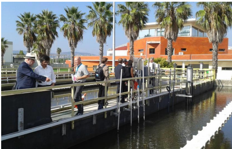
Figure 11: Full Scale Installation Frielas, Portugal
