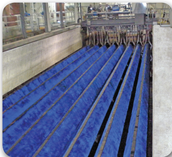
Filter units fitted with the OptiFiber PES-14® microfiber media.
