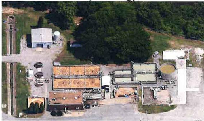
Figure 1. Plant Treating PET Production Wastewater
