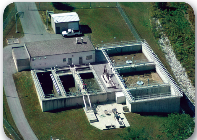
Abbottstown's dual-basin AquaSBR ® system is shown to the right.
