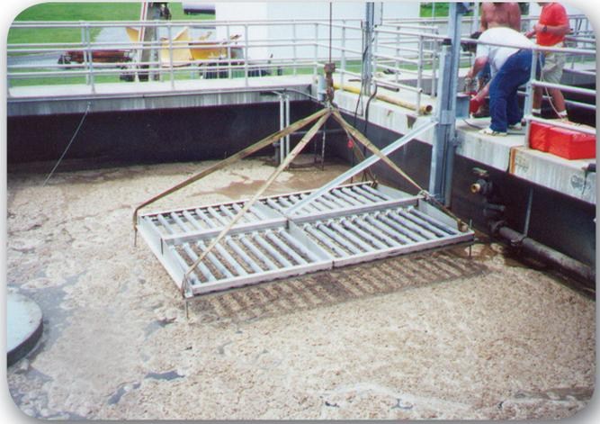
The new fine-bubble assembly on the existing track is being lowered into the basin.
