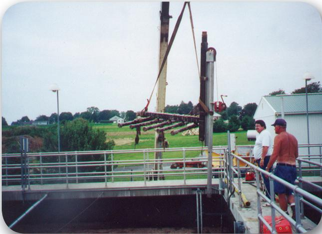
One of the old retrievable coarse-bubble diffuser racks being removed from the basin.
