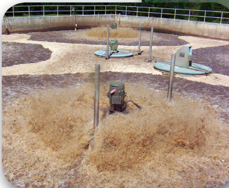
Aerial view showing the 2-basin AquaSBR ® system; a closeup of the system in operation is shown to the left.
