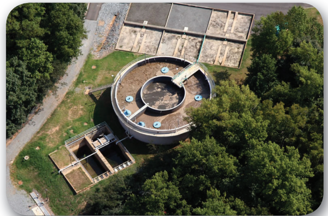
Overview of Warm Spring WWTP's AquaSBR ® system with integral digester in the center. Photo Credit: SblevieProductions
