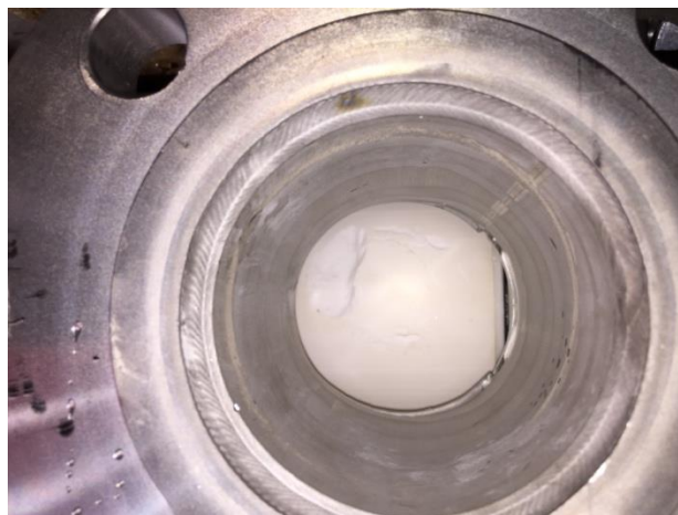
Figure 14 Damage to Ceramic Element
