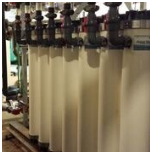
Figure 20. The New Amsterdam Modules with Rerouted Filtrate Piping
